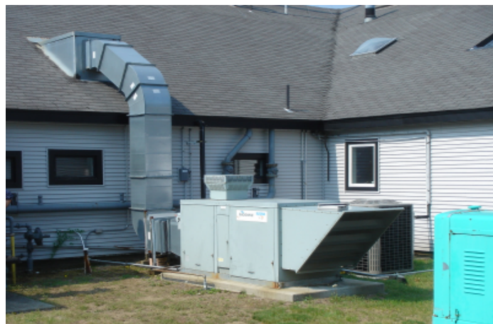
Outdoor Air Handling Unit – Modine Weatherhawk
